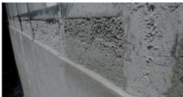
PARTITION WALLS (panels + lightweight concrete)
