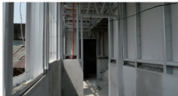
PANEL INSTALLATION (calcium silicate)
