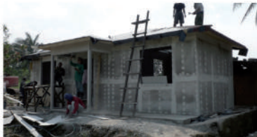
PUTTY APPLICATION (joints and screws)
