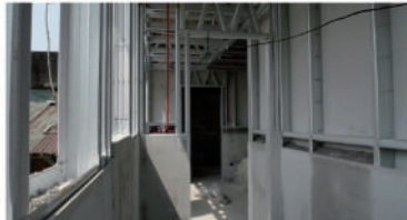
PANEL INSTALLATION (calcium silicate)
