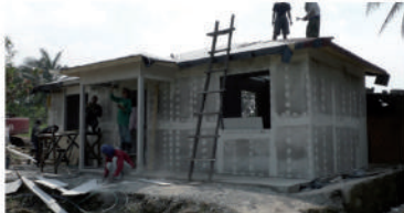
PUTTY APPLICATION (joints and screws)
