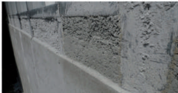
PARTITION WALLS (panels + lightweight concrete)
