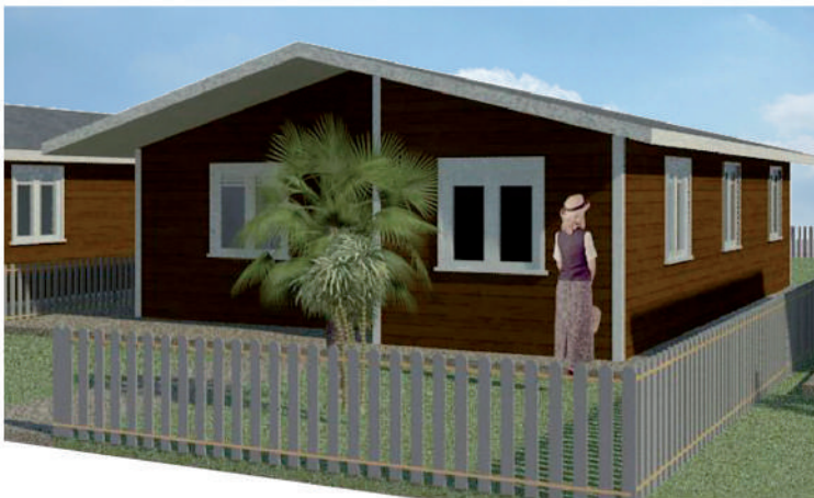
HOUSING EXTERIOR VIEWS
